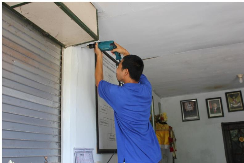
Gambar 4. Pemasangan wifi router
