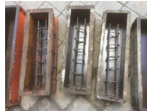
Figure 4. Preparation of pouring fresh concrete
