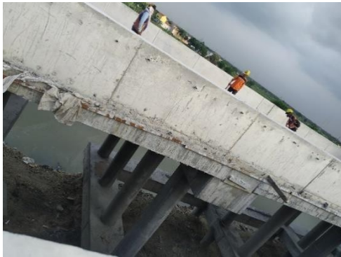
Gambar 1 Sisa Material Geotextile dan Besi Hollow
