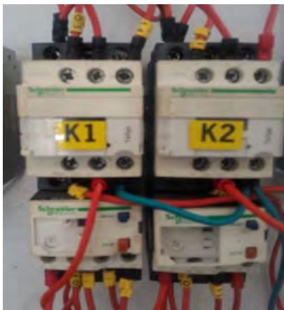
Figure. 8. Contactor and Thermal overload
